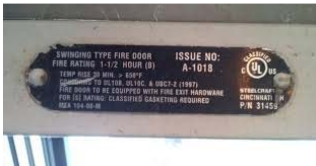
Example of a fire door tag located on the hinge side of the fire door.
